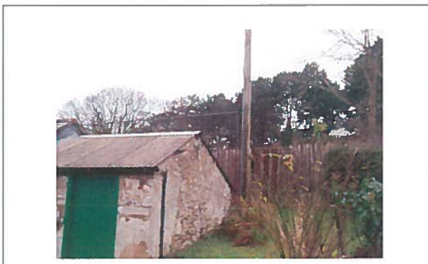
Proposed building plot will be behind fencing of the Bungalow
